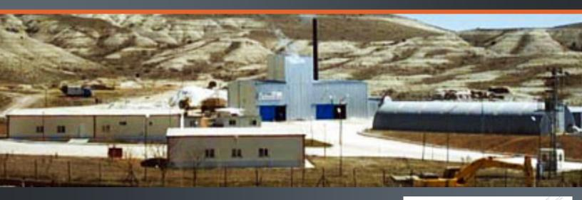
Kazan Soda Maden Enerji Nakliyat Sanayi Ve Tic A.Ş. A.Ş (Kazan Soda) is owned by Ciner Holding one of the largest Turkish conglomerate groups. This greenfield project involves the construction of a new Dense Soda Ash and Sodium Bicarbonate Process Plant in the Kazan Province of Turkey, approximately 35 km North-West of Ankara. The project will use solution mining to extract the ore. Ciner Holding owns the mining license for the Natural Trona Mine Area.
